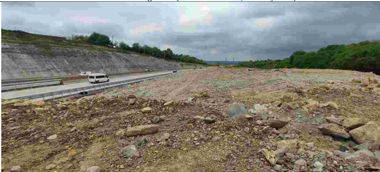
Temporary Spoil Storage (Near Tunnel Portal 5 - Argveta Site, May 2024)
