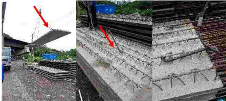
Picture 3: Positive and Negative observation – Lifting safety (All tunnel and bridges) – Good and bad (Including handmade) quality lifting equipment has been observed during site inspection. The Engineer has asked the Contractor's site responsible persons to take care of this issue and pay additional attention at to avoid the possible incidents and injury of working personnel. Issue isn't solved yet.
