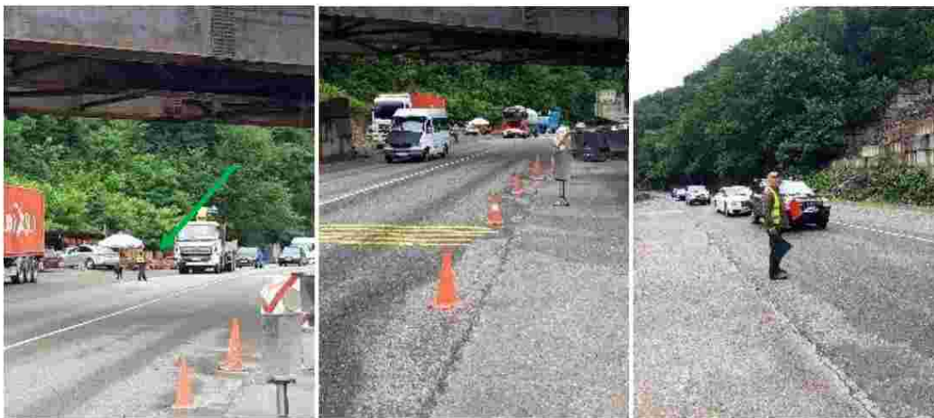
Picture 13: Positive Observation – Lifting safety (Main road (E60)) – Safe lifting process has been observed during site inspection. It has been observed that the working area was protected by using traffic flash cones and plus, the flagmen were appointed to control the movement of the vehicles crossing the workplace.
