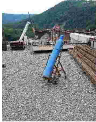
Workshop (Bridge N2)
