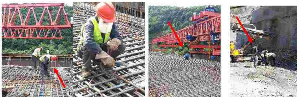
Bridge N1 TA
