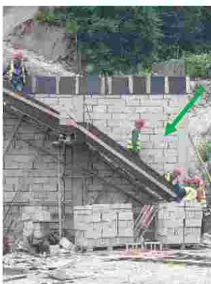
Tunnel portal N3AT-A
