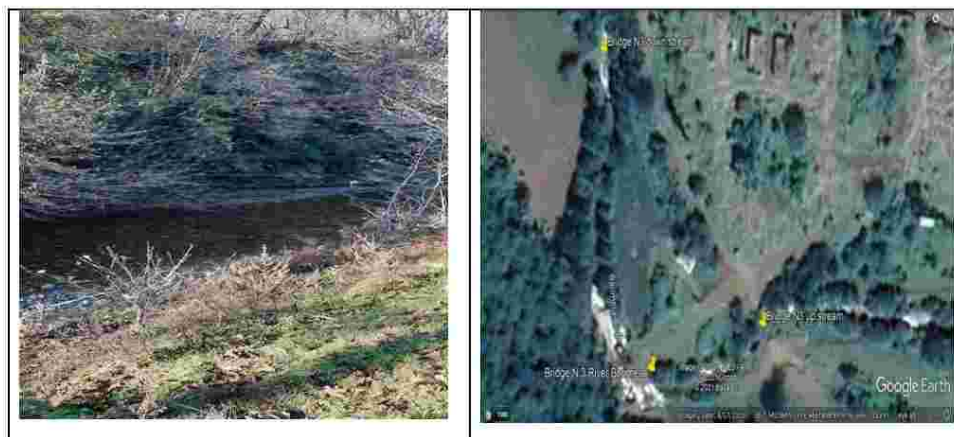
Figure 5-2 Bridge N3 downstream (Borimela River)
