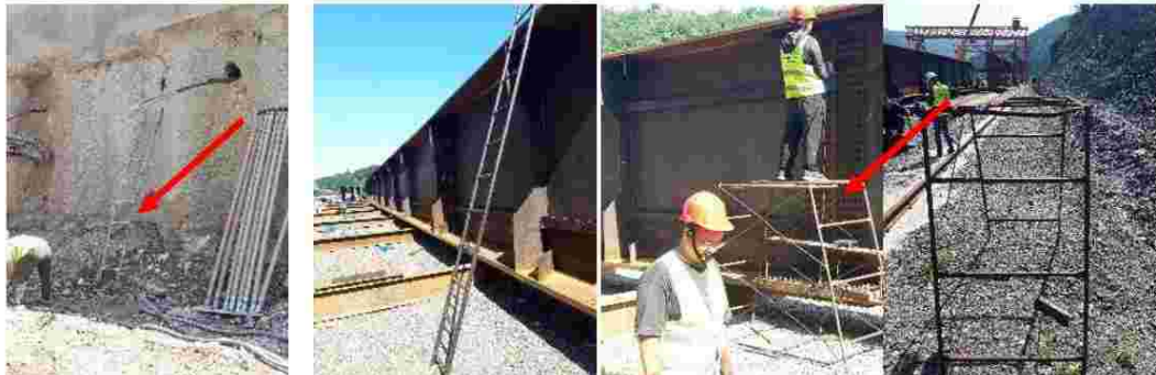
Tunnel N 1 (Argveta side)
