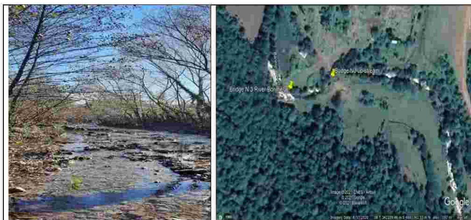
Figure 5-1 Bridge N3 upstream (Borimela River)
