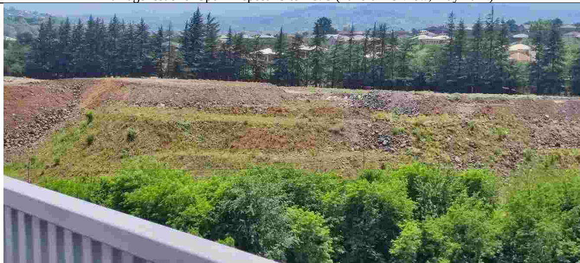
Spoil Disposal Site No: 2 (Panoramic View, May 2024)
