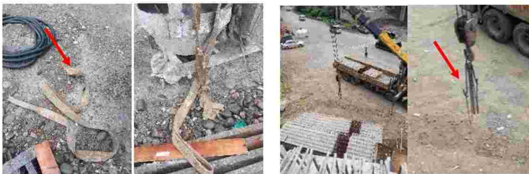
Tunnel N1 AT (Argveta side)
